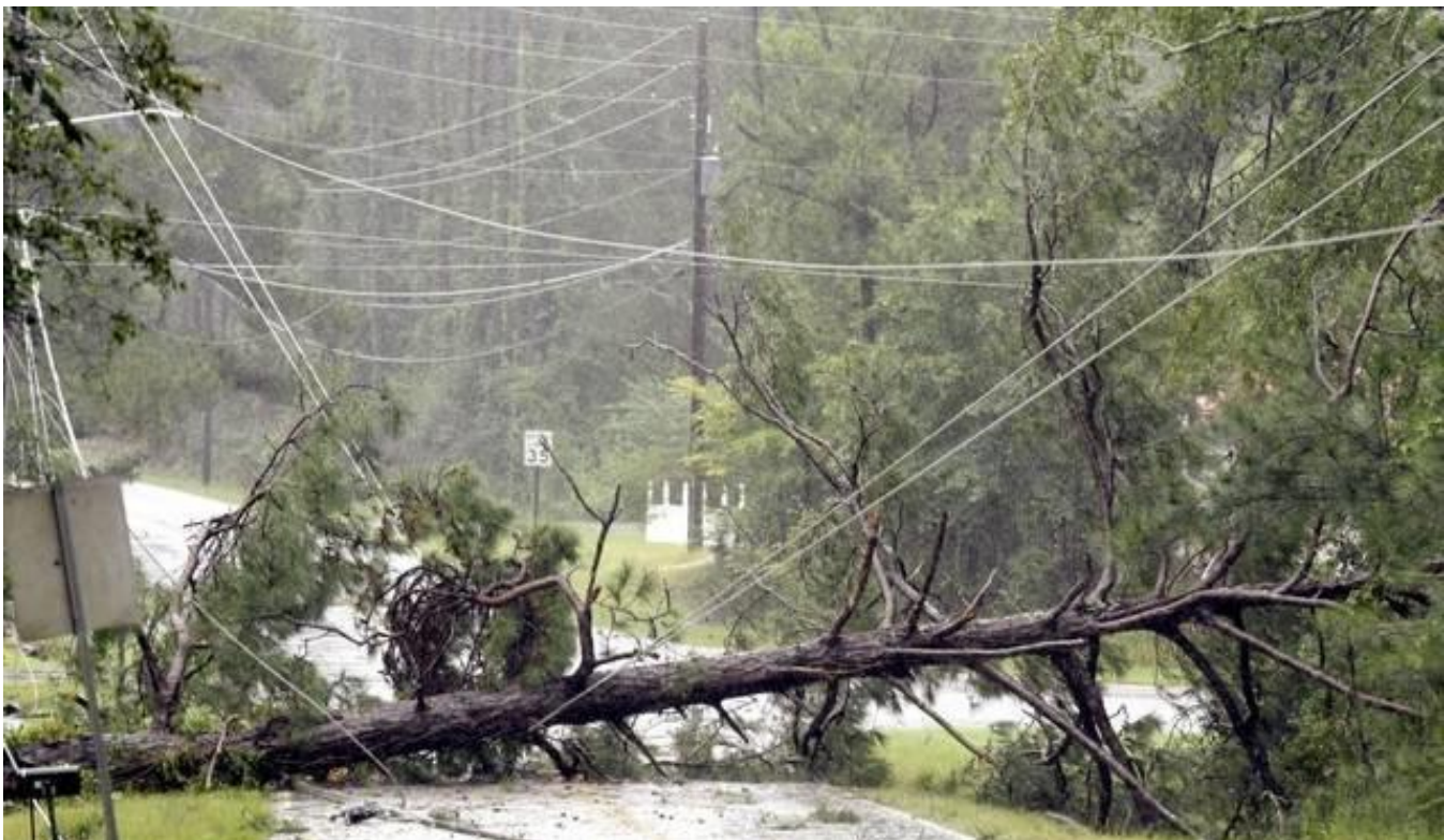
Figure 9.12: Damage in Macon, Georgia
