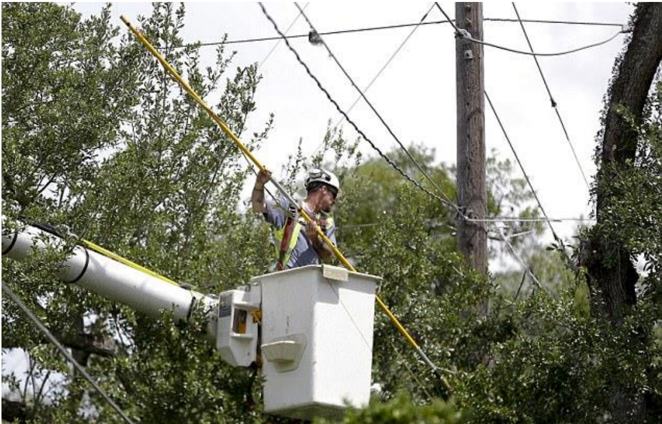
Figure 9.11: Clearing vegetation in Orlando, Florida
