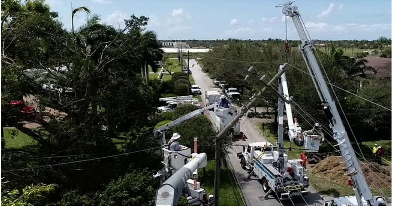
Figure 9.13: Restoration in Progress
