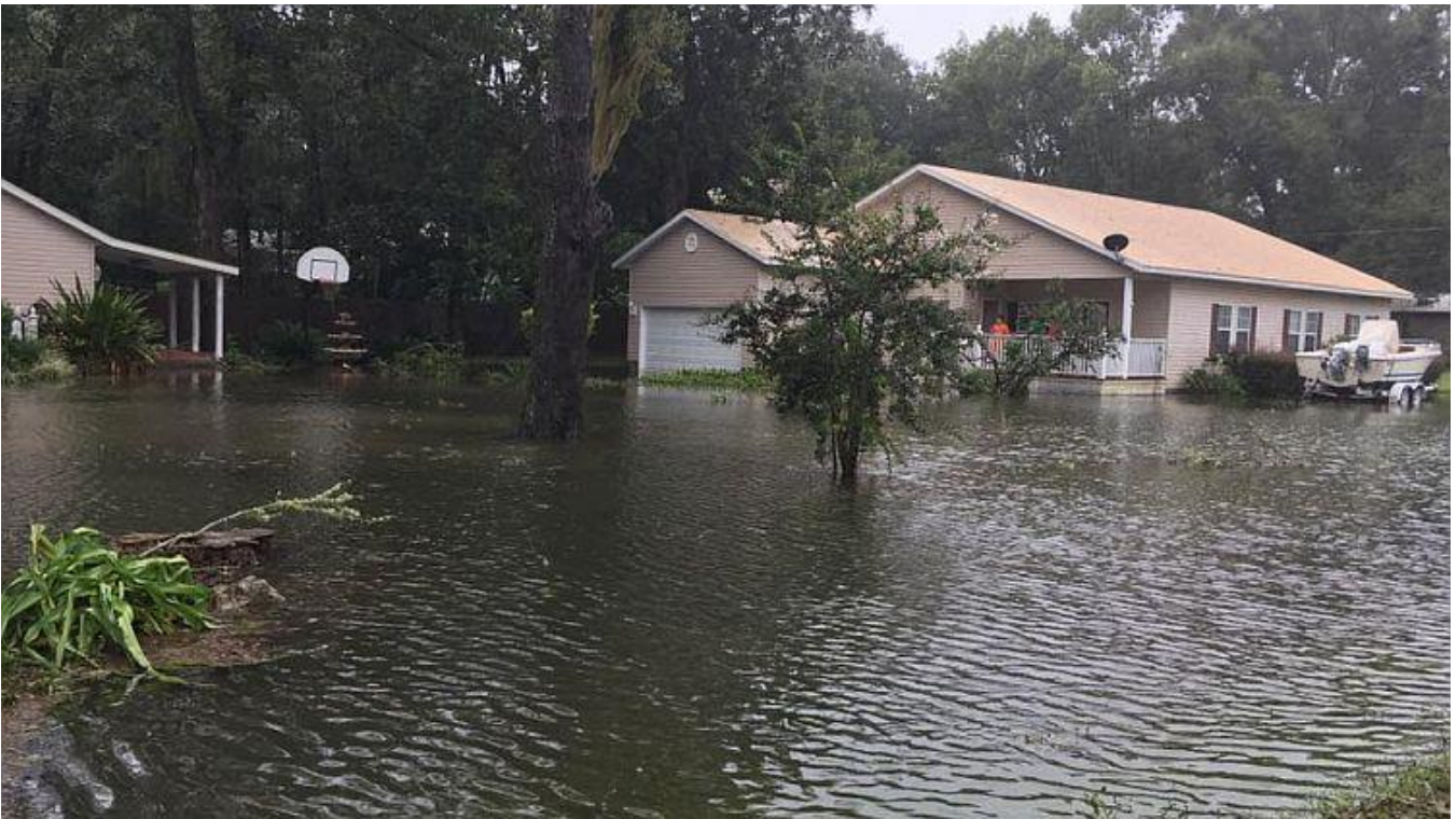
Figure 9.6: Flooding in Alachua—North Central Florida
