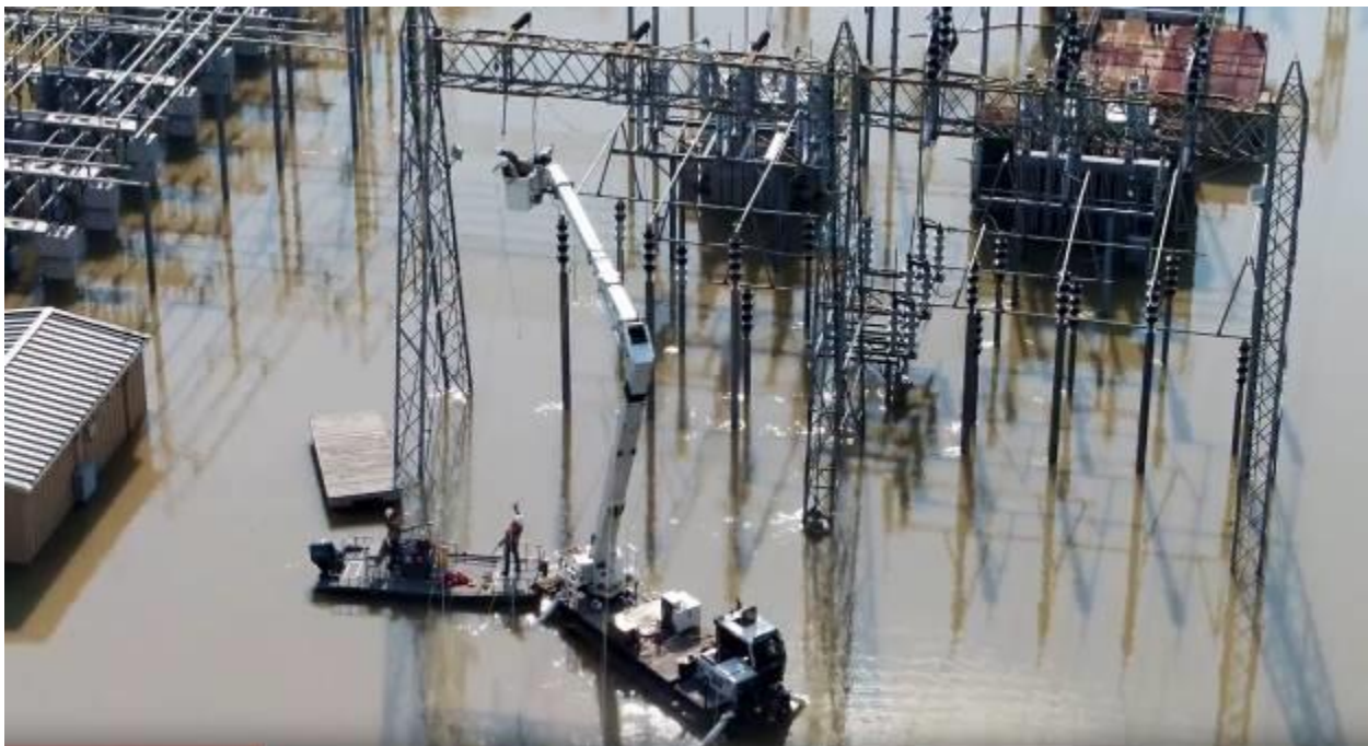
Figure 10.6: Flooded substation
