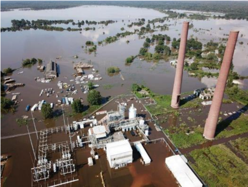
Figure 10.7: Flooded power plant
