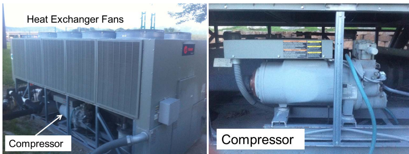
Figure 10: Three-Phase Motors Outside Hotel in Salt Lake
